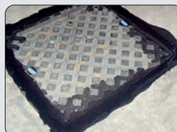
Scellage des cockpits
