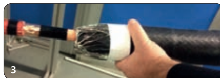
3 Position at the centre of the connection and collapsed on the cable removing the inner support
