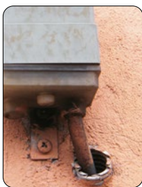
Corrugated pipe entry protection
