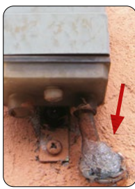
Corrugated pipe entry protection
