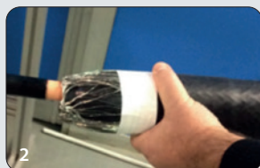
2 The joint is fitted on the connected cable.
