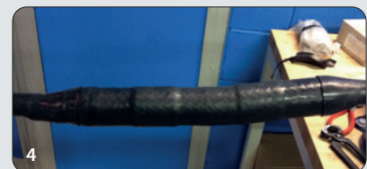
4 The joint is completed and can be used immediately.
