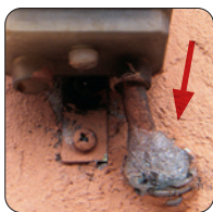
Corrugated pipe entry protection
