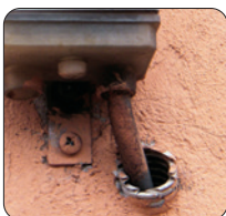
Corrugated pipe entry protection
