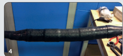
4 The joint is completed and can be used immediately.
