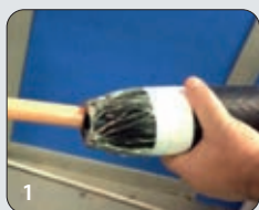
1 The body of the joint carries the integrated shield and outer sheath.
