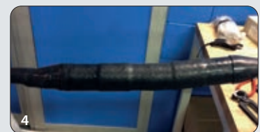
4 The joint is completed and can be used immediately.
