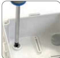
Fix the box and cover the screws with the caps.
