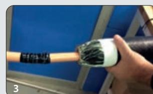
Position at the centre of the connection and collapsed on the cable removing the inner support.
