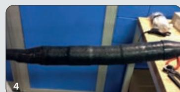
The joint is completed and can be used immediately.
