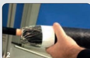
The joint is fitted on the connected cable.
