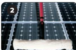
Let stand for a few minutes, depending on the level of dirt to be cleaned, then wipe with a soft, non-abrasive, slightly damp pad or sponge.
