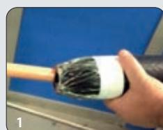
The body of the joint carries the integrated shield and outer sheath.
