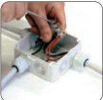
Insert the cables and connect the wires.
